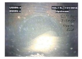
Tile in the upper end on the west side of the tracks. Shows round but with silt and debris.
